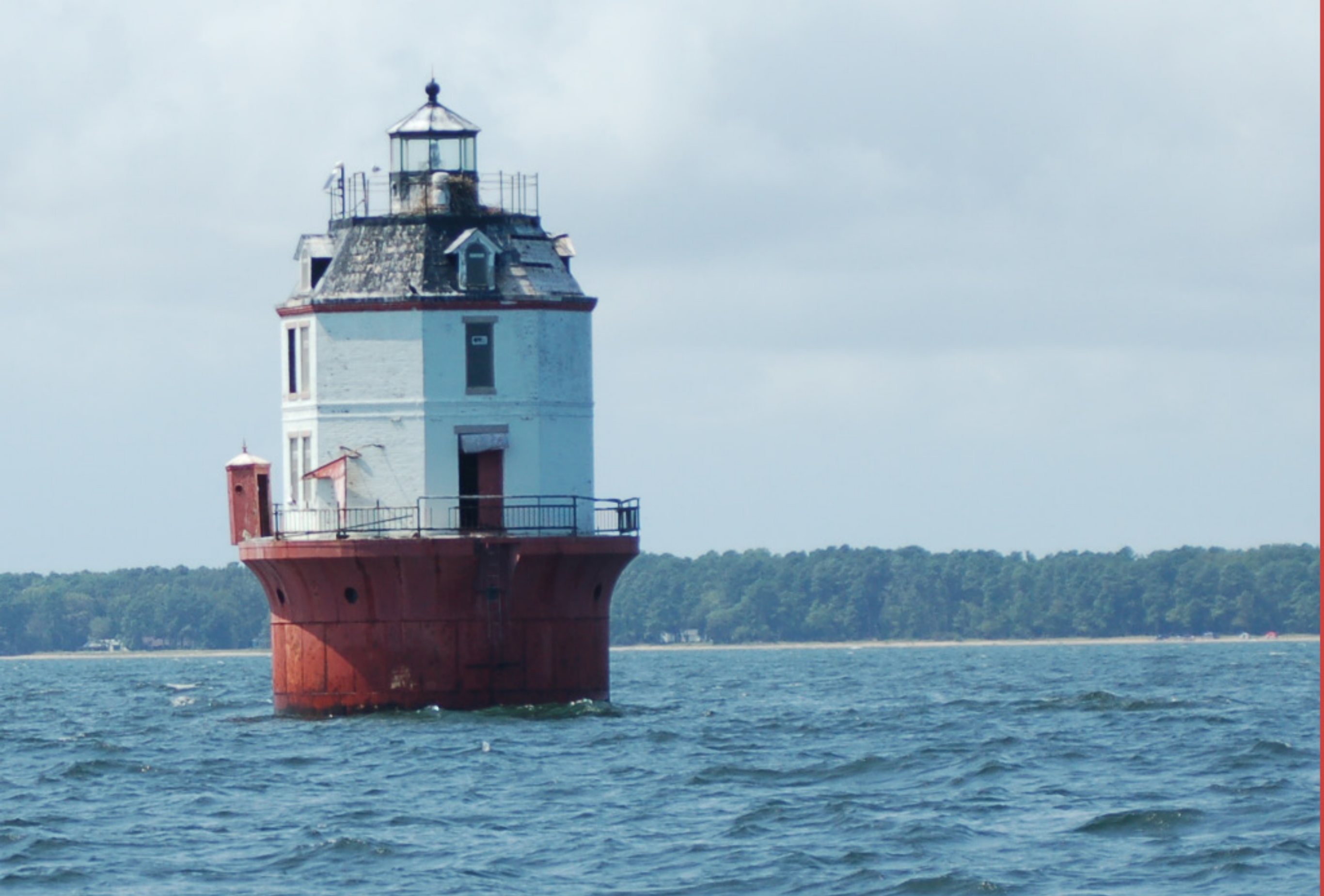
Smith Point Light, well ventilated out house, entrance Potomac River
